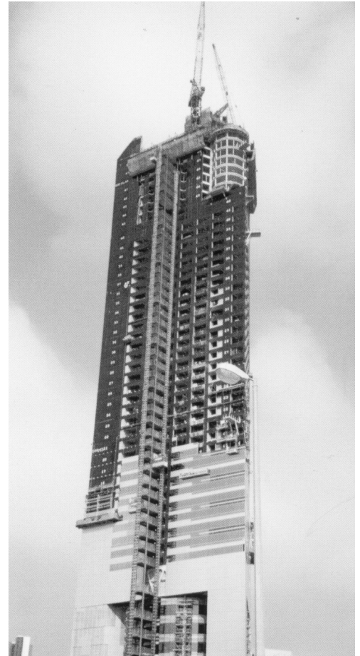
Emirate Twin Tower Project, Tower TP10. Tallest building in the Middle East - fireproofed with Cafco 300
